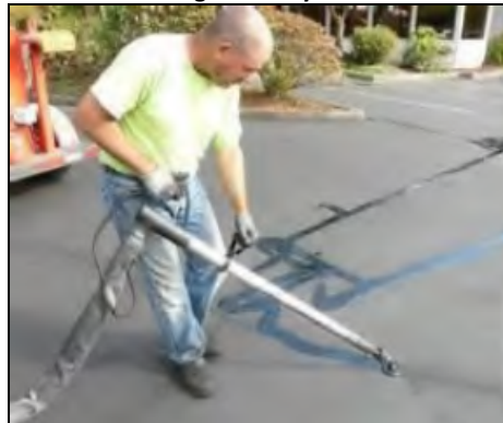
Sealing Roadway Cracks
