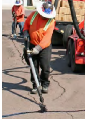
Crack Sealing
