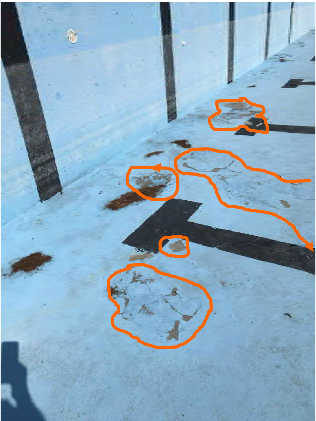
Broad areas of spalling and delamination
