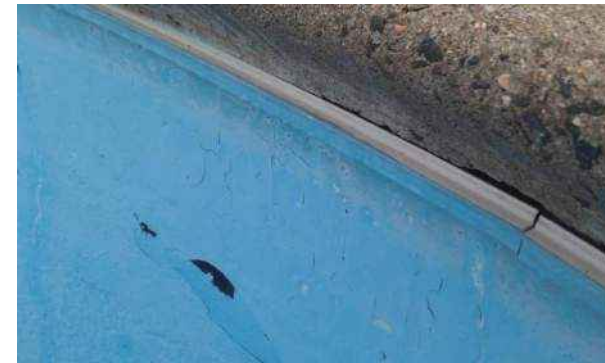
Figure 6 – Peeling paint and PVC joint separation
