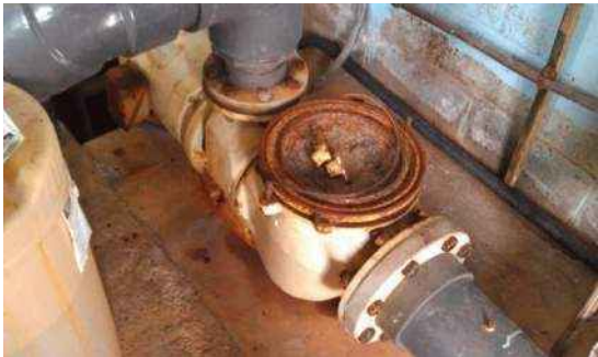
Figure 19 – Main pool pump
