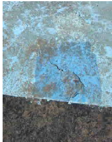
Previously repaired areas in pool floor with failure of repair materials
