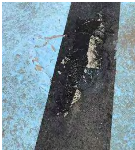
Previously repaired areas in pool floor with failure of repair materials
