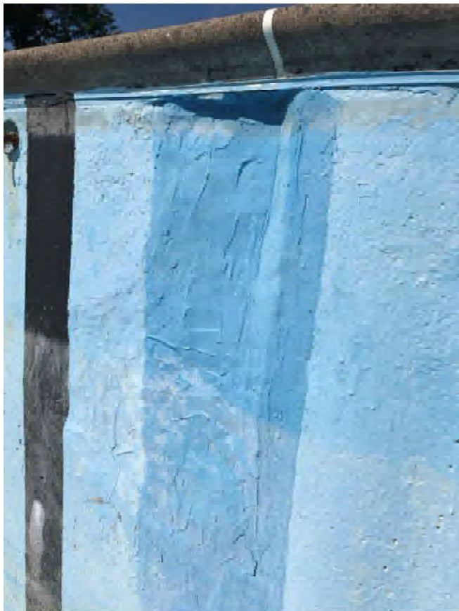
Significant spall of approximately 4-inches deep
