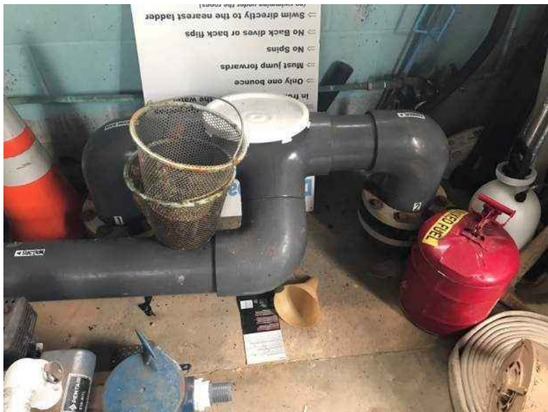
Above: 10 HP recirculation pump. Below Right: Main drain and skimmer suction piping. Below Left: Pump discharge to Filters
