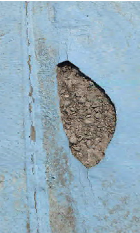
Delamination adjacent to construction joint
