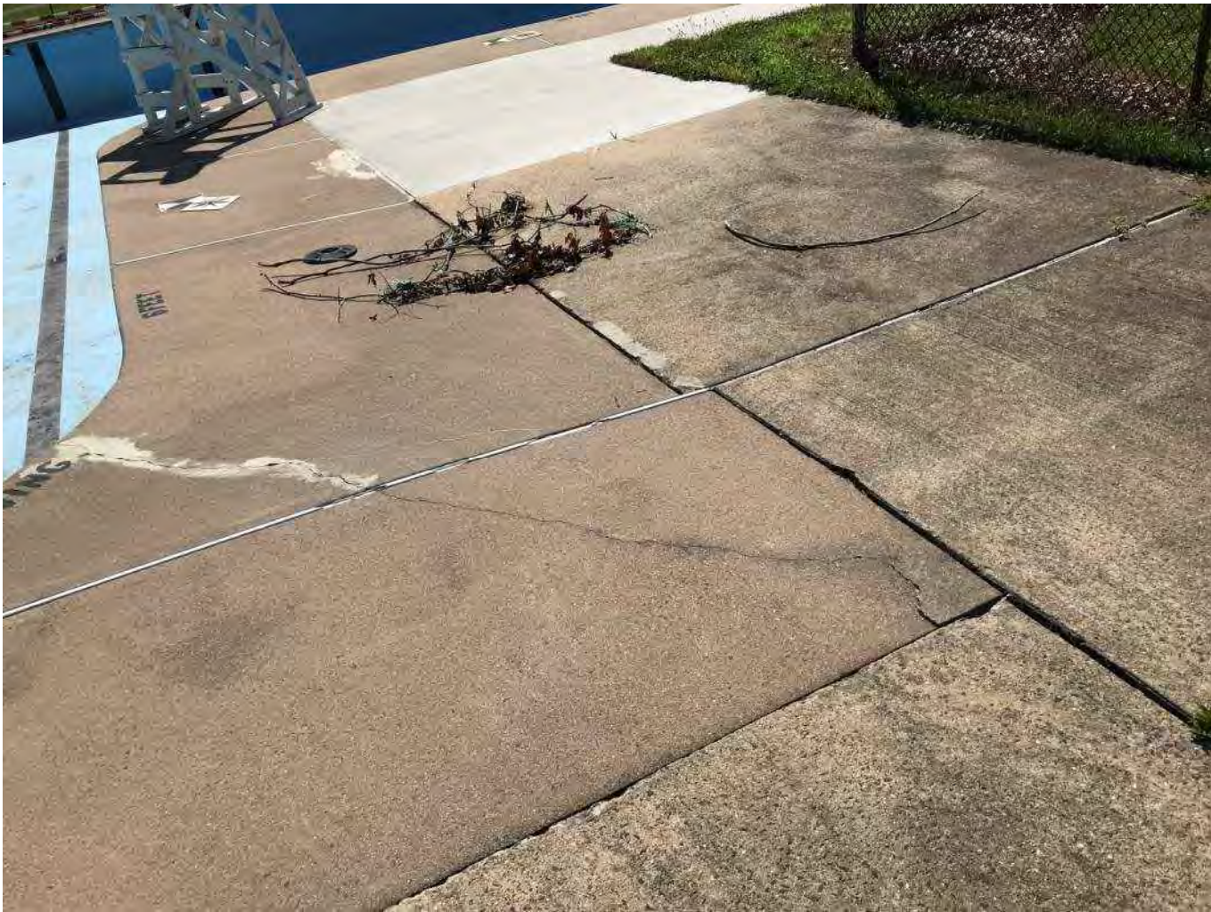
Typical deck conditions. Note 1990's vintage decking closest to pool, original decking in foreground and recently replaced decks toward the back of the photo. 1990's vintage decking is generally in good condition, though there are some significant cracks and areas of damage. Differential settlement has also caused misalignments and failed sealant joints exacerbates freeze/thaw damage.
