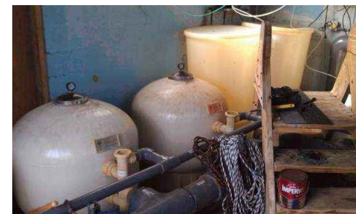
Figure 17 – Main pool filters, chemical storage, and stairs
