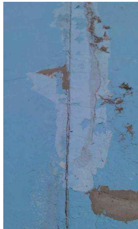
Figure 5 – Expansion joint, cracks, and patches
