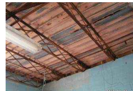
Figure 29 – Original steel roof structure of filter building
