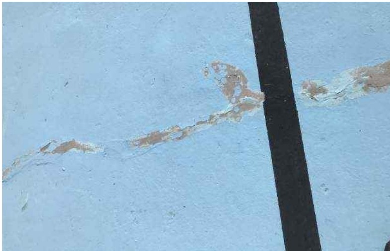
Previously repaired crack in pool floor with failure of repair materials
