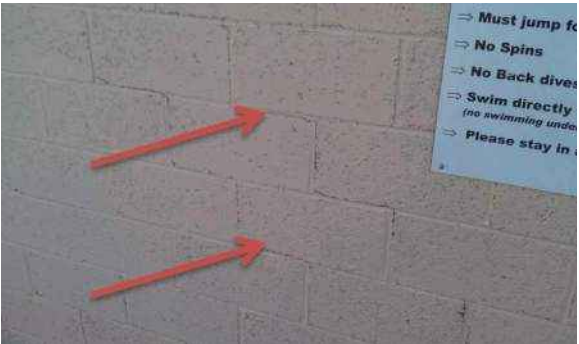
Figure 22 – Traveling cracks on filter building
