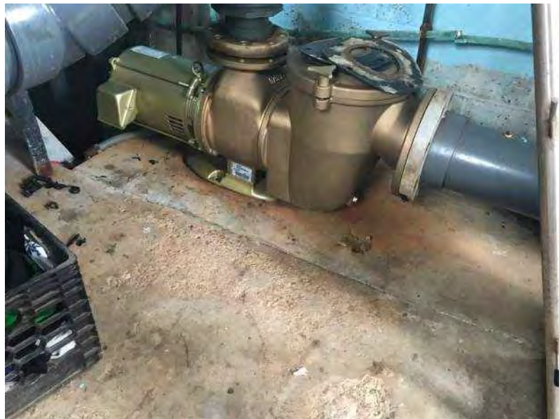
Above: 10 HP recirculation pump. Below Right: Main drain and skimmer suction piping. Below Left: Pump discharge to Filters
