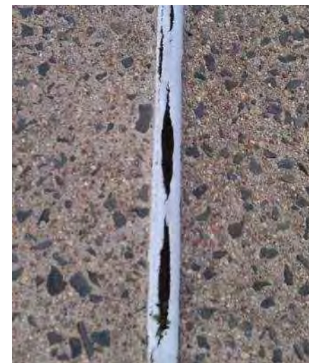
Figure 7 – Failed expansion joint caulking
