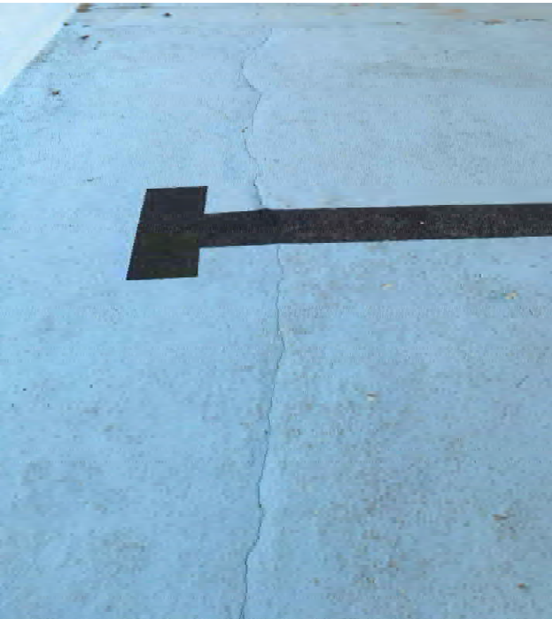
Typical crack in pool floor
