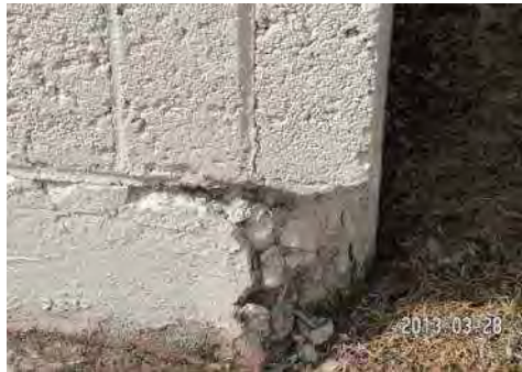
Figure 31 – Foundation spalling
