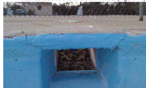
Figure 14 – Wading pool cracked coping above skimmer
