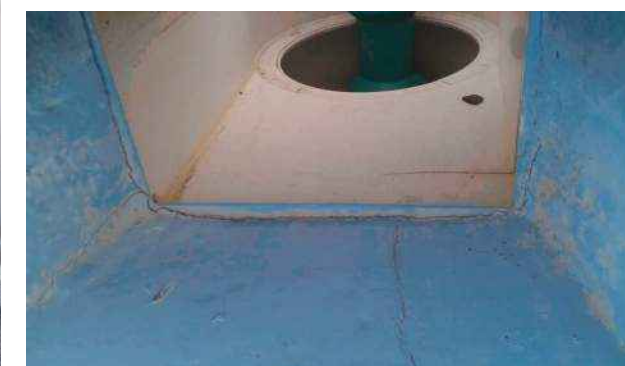
Figure 13 – Cracked joint between concrete and skimmer
