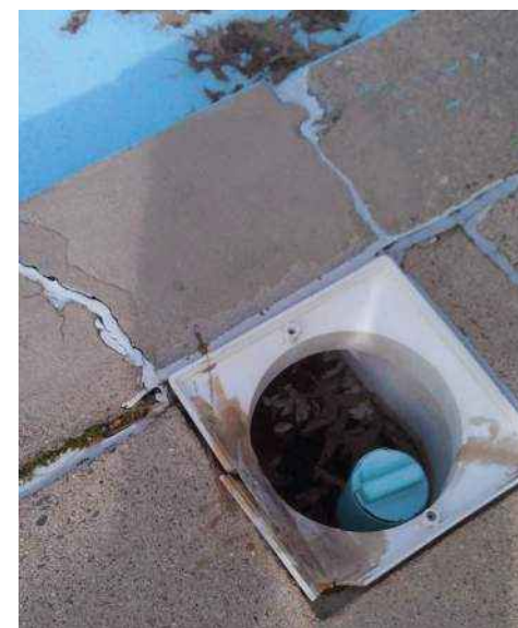
Figure 15 – Cracked skimmer and coping concrete
