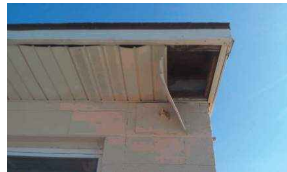
Figure 28 – Soffit and fascia damage
