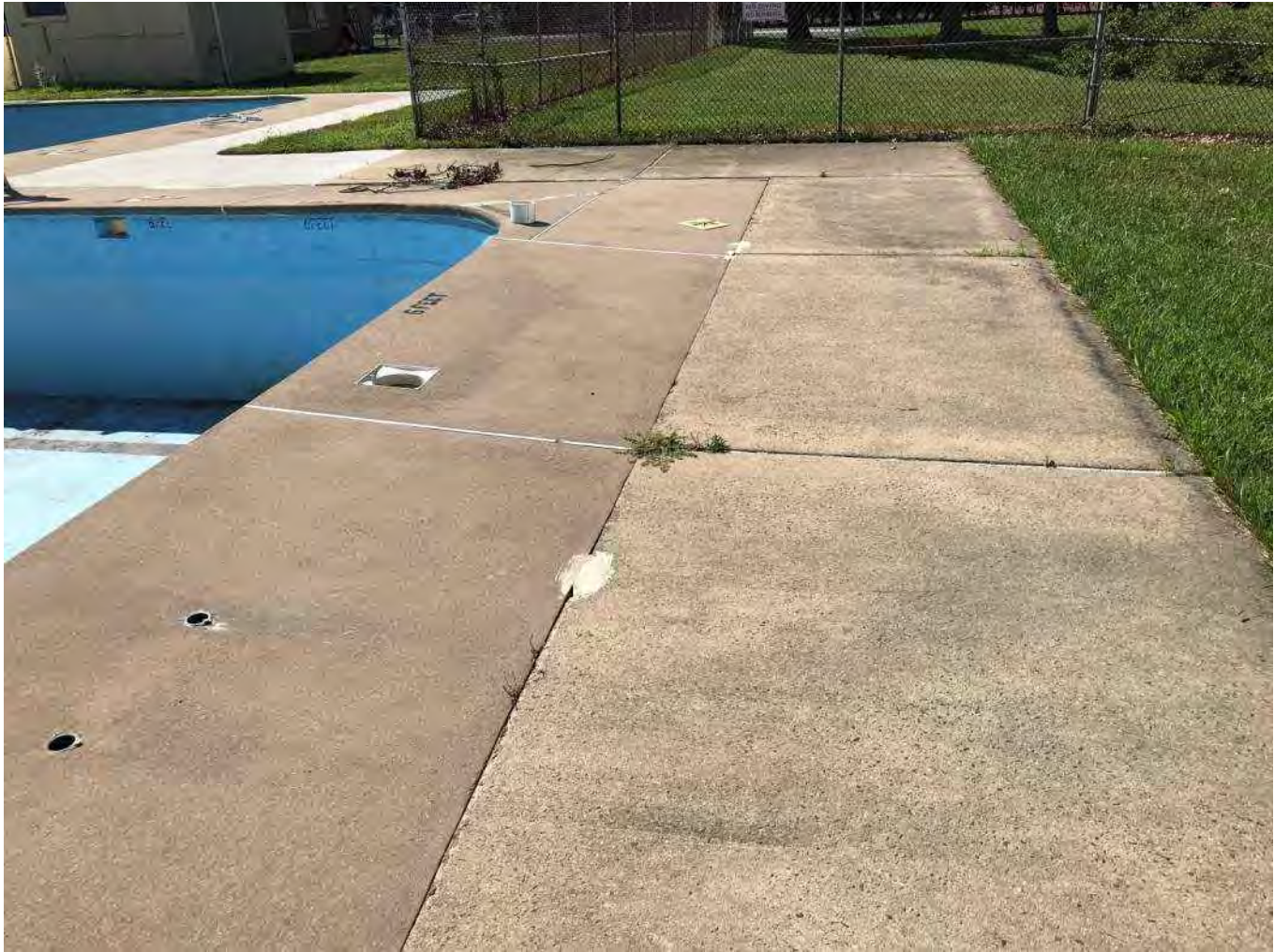
Deck pitch at the slab adjacent to the pool exceeds the ADA allowable cross pitch of 1:48. This maximum slope must be maintained for an accessible route from the bathhouse to the HCA Lift Chair and the Steps.
