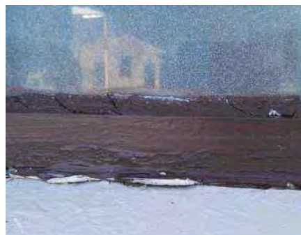
Figure 27 – Window glazing failure
