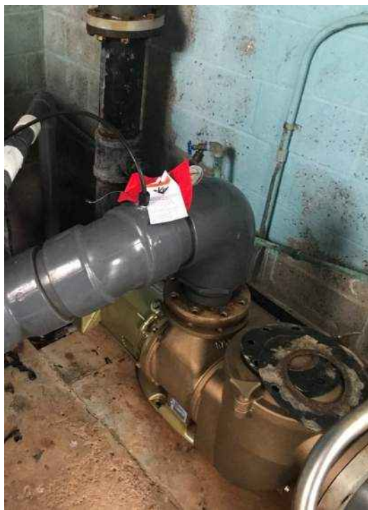
Above: 10 HP recirculation pump. Below Right: Main drain and skimmer suction piping. Below Left: Pump discharge to Filters
