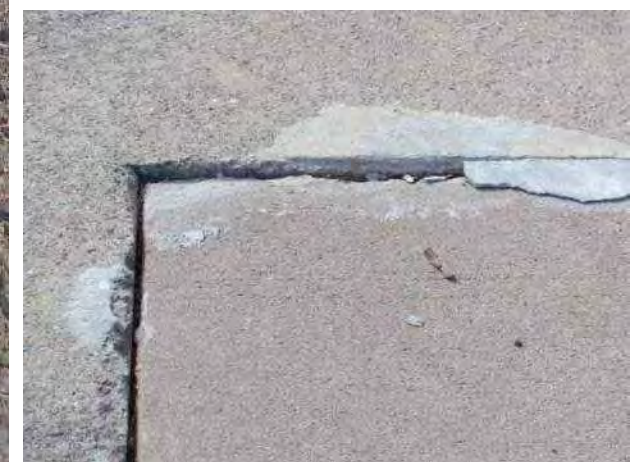
Figure 8 – Frost heave or settling concrete deck
