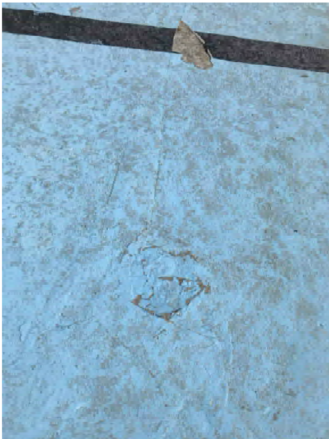
Multiple delaminations along the edge of crack
