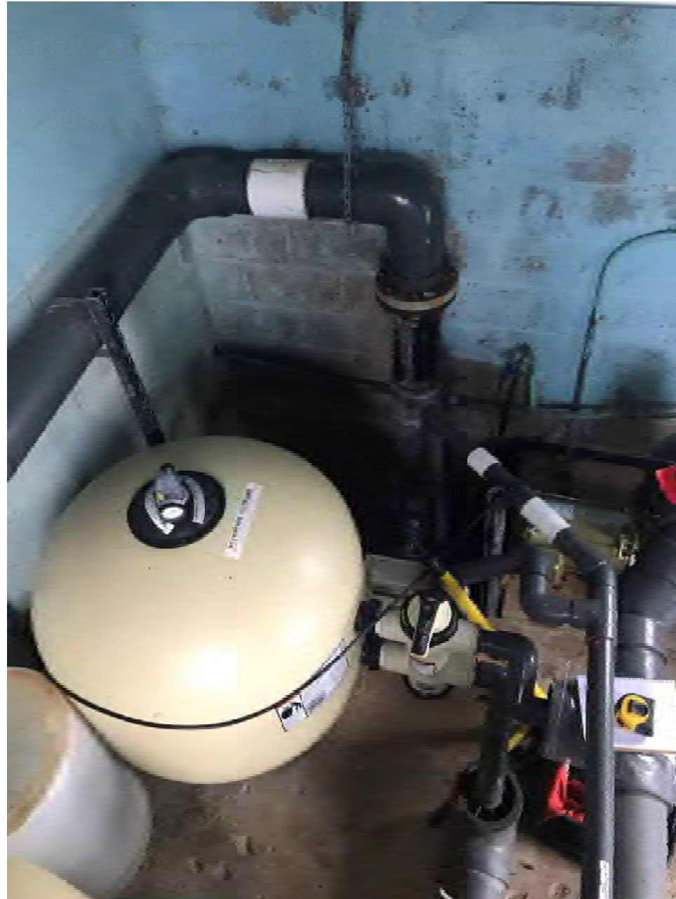
Typical filter piping and multi-port valve. Position of the valve determines filter mode –vs– backwash mode.
