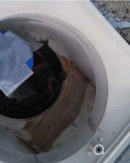
Figure 12 – Repaired skimmer
