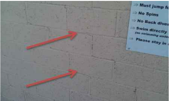
Figure 22 – Traveling cracks on filter building
