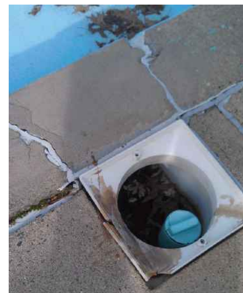
Figure 15 – Cracked skimmer and coping concrete
