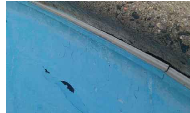
Figure 6 – Peeling paint and PVC joint separation
