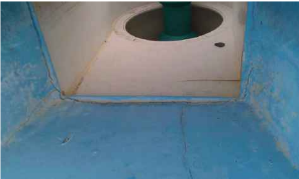
Figure 13 – Cracked joint between concrete and skimmer
