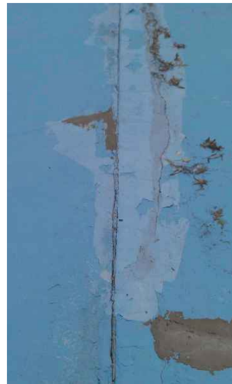
Figure 5 – Expansion joint, cracks, and patches
