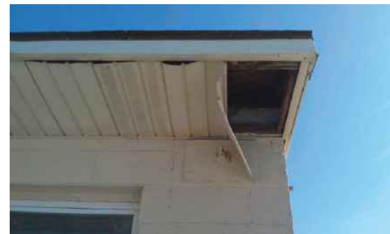
Figure 28 – Soffit and fascia damage
