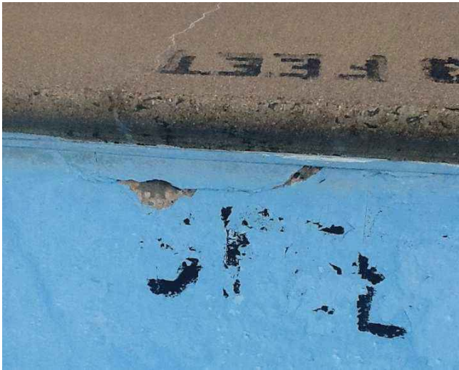
Figure 9 – Peeling depth markers
