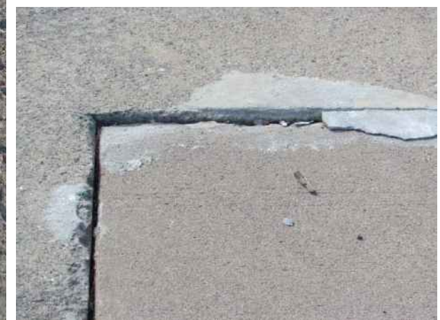
Figure 8 – Frost heave or settling concrete deck
