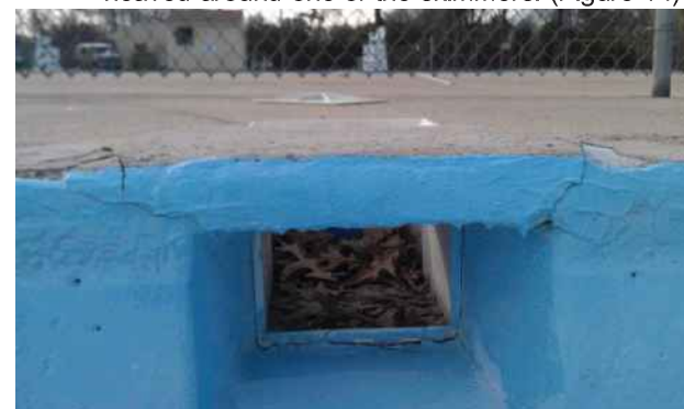
Figure 14 – Wading pool cracked coping above skimmer
