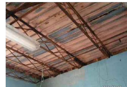
Figure 29 – Original steel roof structure of filter building
