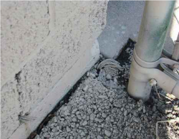
Figure 18 – Cut bonding or grounding wire
