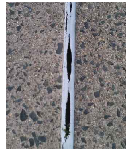
Figure 7 – Failed expansion joint caulking
