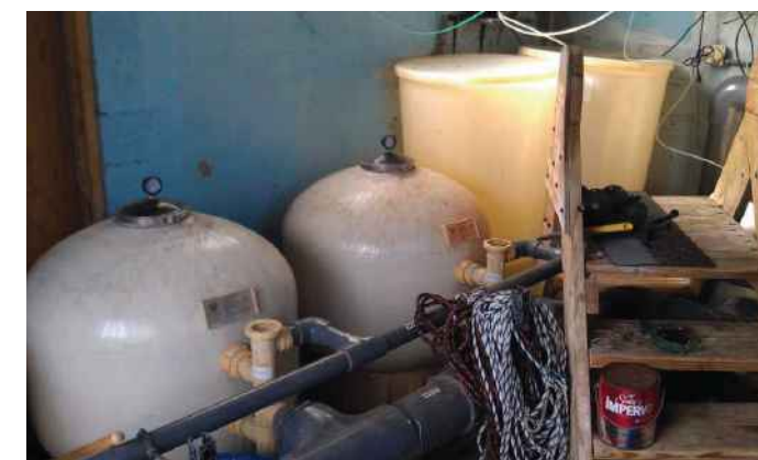
Figure 17 – Main pool filters, chemical storage, and stairs
