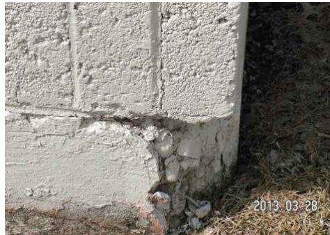
Figure 31 – Foundation spalling
