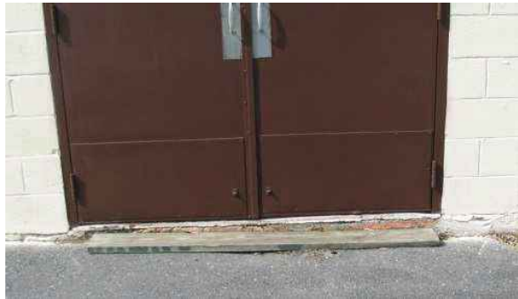
Figure 32 – Bathhouse entrance trip hazard
