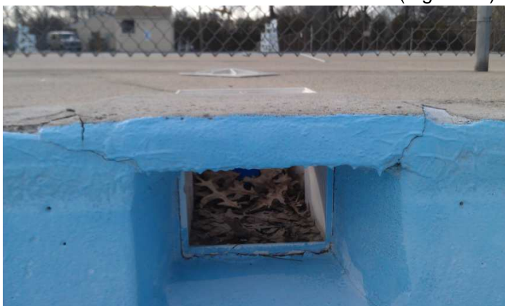
Figure 14 – Wading pool cracked coping above skimmer
