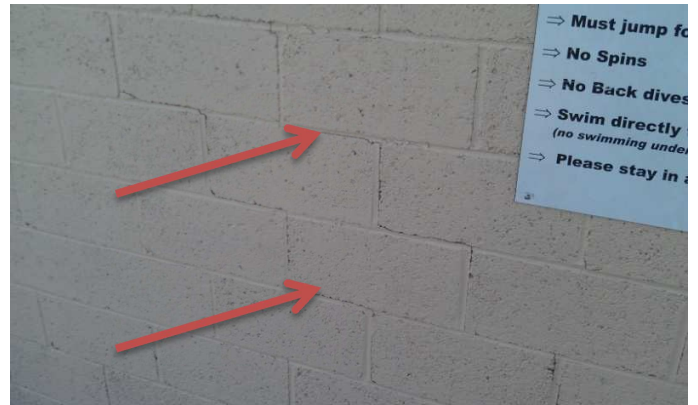
Figure 22 – Traveling cracks on filter building
