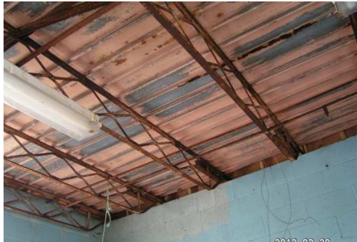
Figure 29 – Original steel roof structure of filter building
