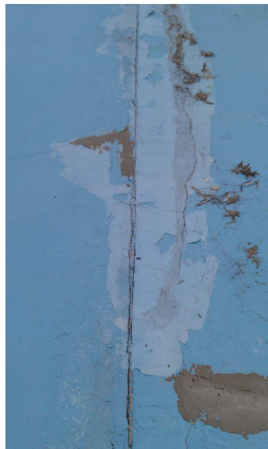
Figure 5 – Expansion joint, cracks, and patches
