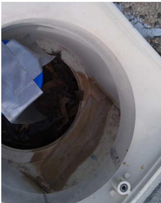
Figure 12 – Repaired skimmer
