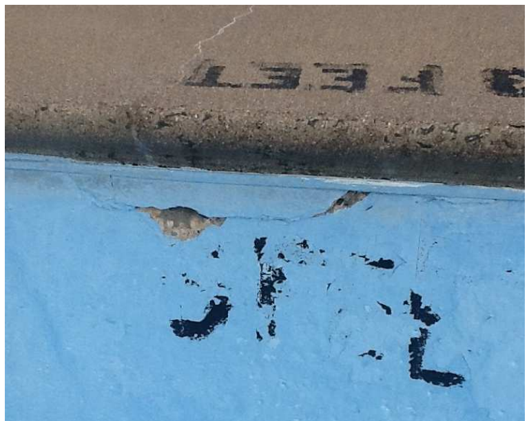
Figure 9 – Peeling depth markers
