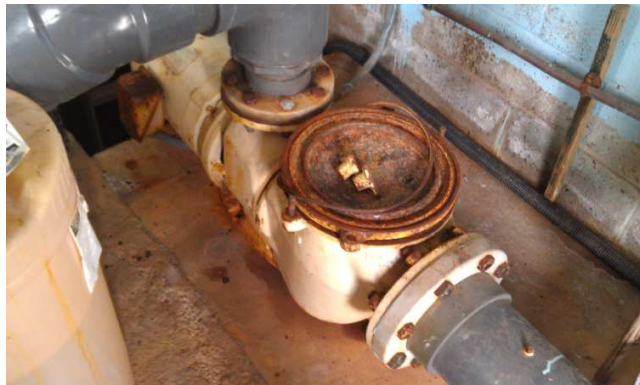
Figure 19 – Main pool pump
