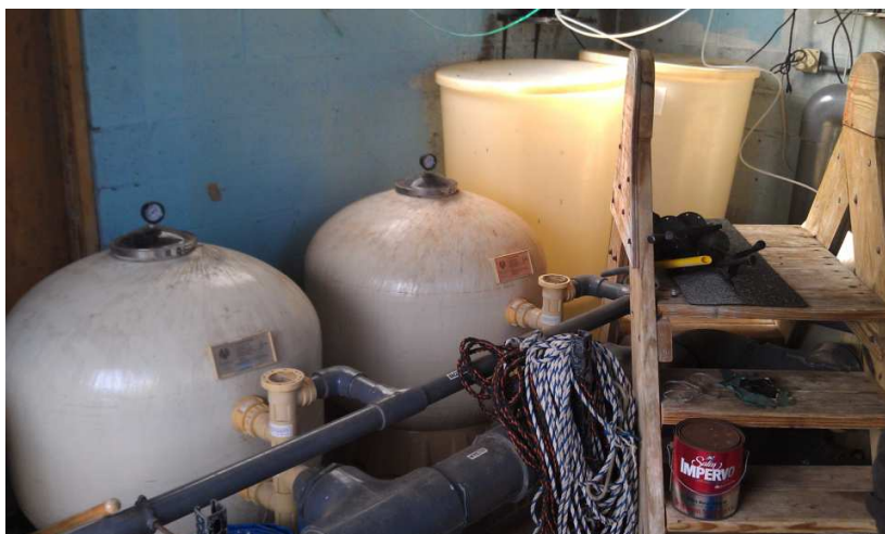
Figure 17 – Main pool filters, chemical storage, and stairs
