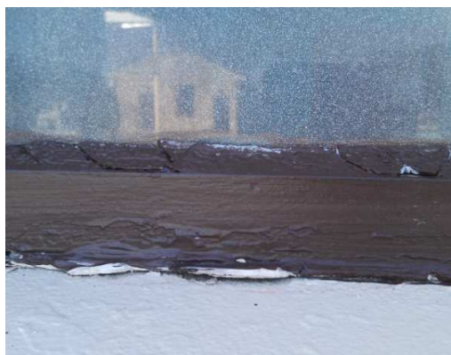
Figure 27 – Window glazing failure
