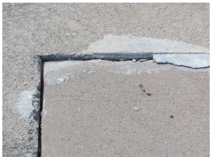
Figure 8 – Frost heave or settling concrete deck
