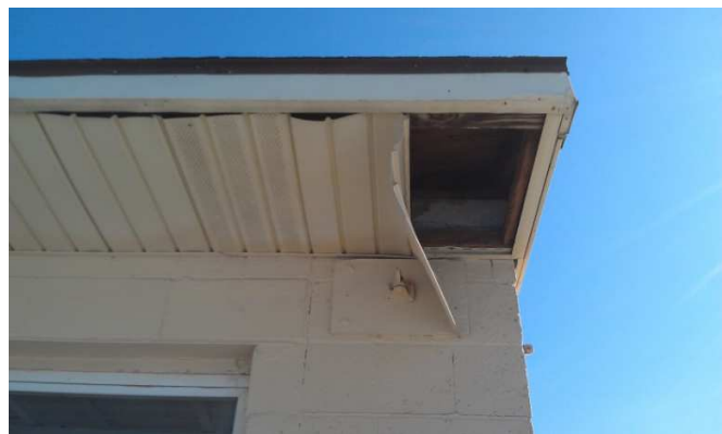
Figure 28 – Soffit and fascia damage
