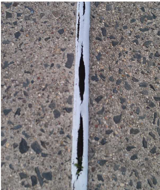
Figure 7 – Failed expansion joint caulking
