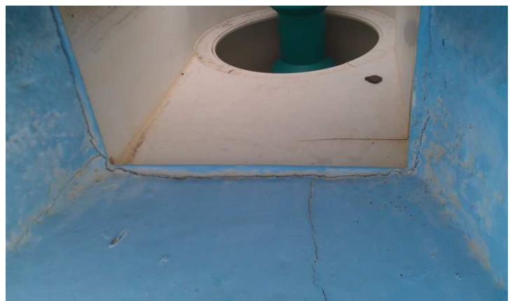
Figure 13 – Cracked joint between concrete and skimmer
