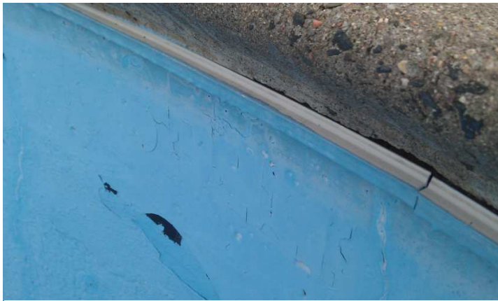
Figure 6 – Peeling paint and PVC joint separation
