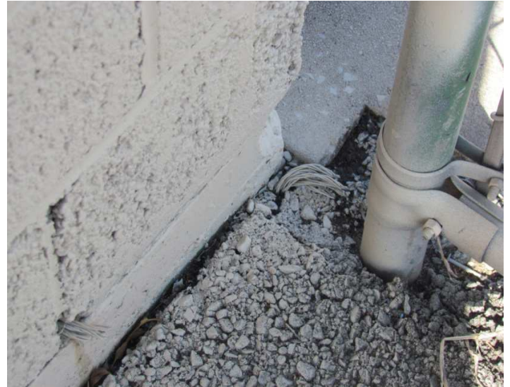
Figure 18 – Cut bonding or grounding wire
