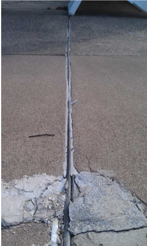
Figure 11 – Copper pipe for handicap lift
