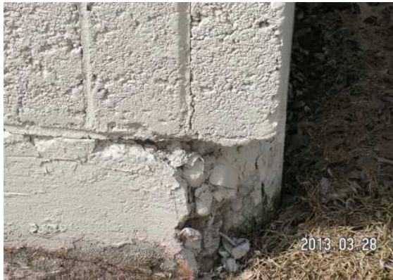
Figure 31 – Foundation spalling
