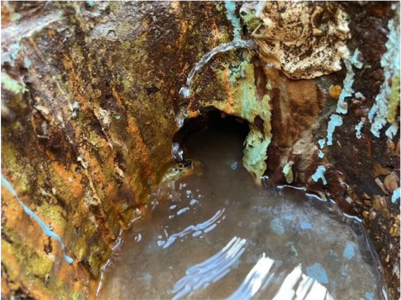
Mill Pond Leaking Sump:
