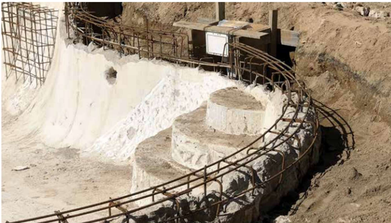
Figure 4: Pool Renovation with Concrete (shotcrete.org)
