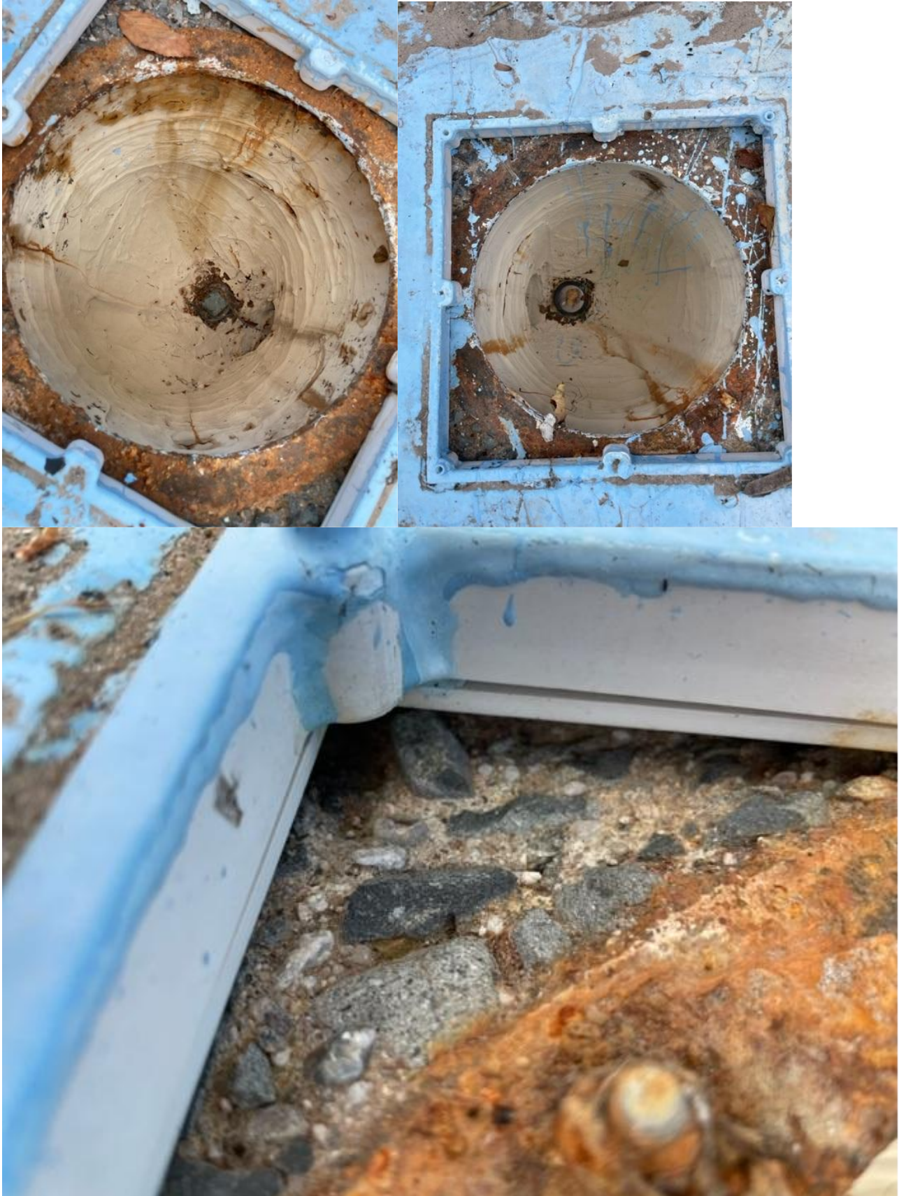
Churchill Failing Fiberglass Coating in Sump and water loss locations:
