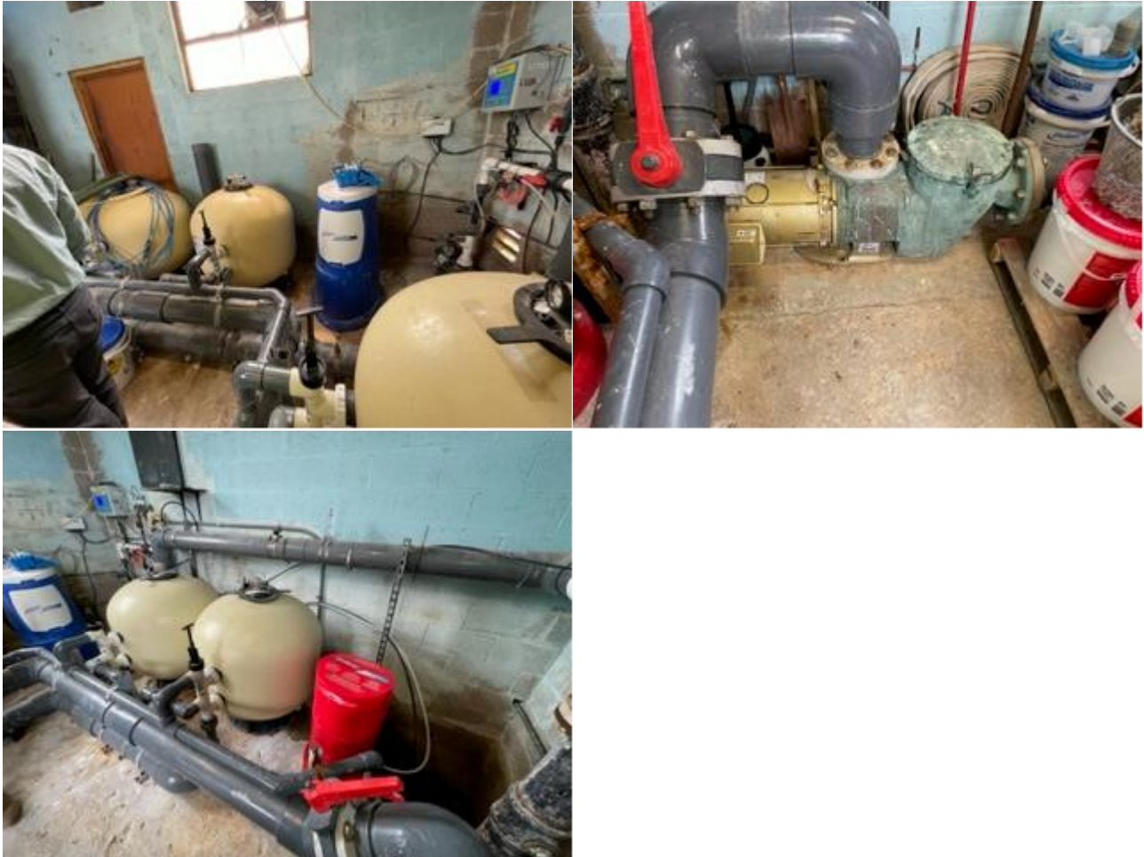
Mill Pond Filters and Pump:
